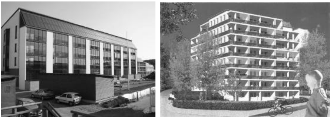
Figure 4. Left: One of the solar heating systems (solar roof) in Ekoviikki. Right: PV balcony in Ekoviikki.
