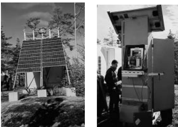
Figure 5. Solar hydrogen systems developed in Finland for stand-alone remote applications.
